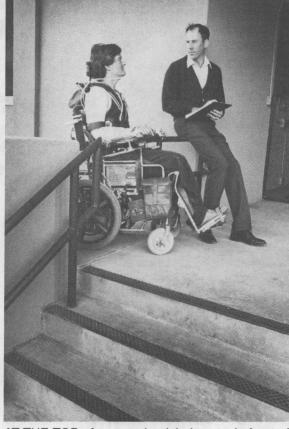
AT THE TOP of a new wheelchair ramp in front of Bldg. 836, Blase Gaude (5021, left) and Wayne Burton (7845) discuss recent facilities work that has improved accessibility to the building for people with disabilities. A sensor above the ramp triggers automatic foyer doors, and a button inside the building opens the doors as well. Before the new ramp was installed, the steps in the foreground were major obstacles for employees with
